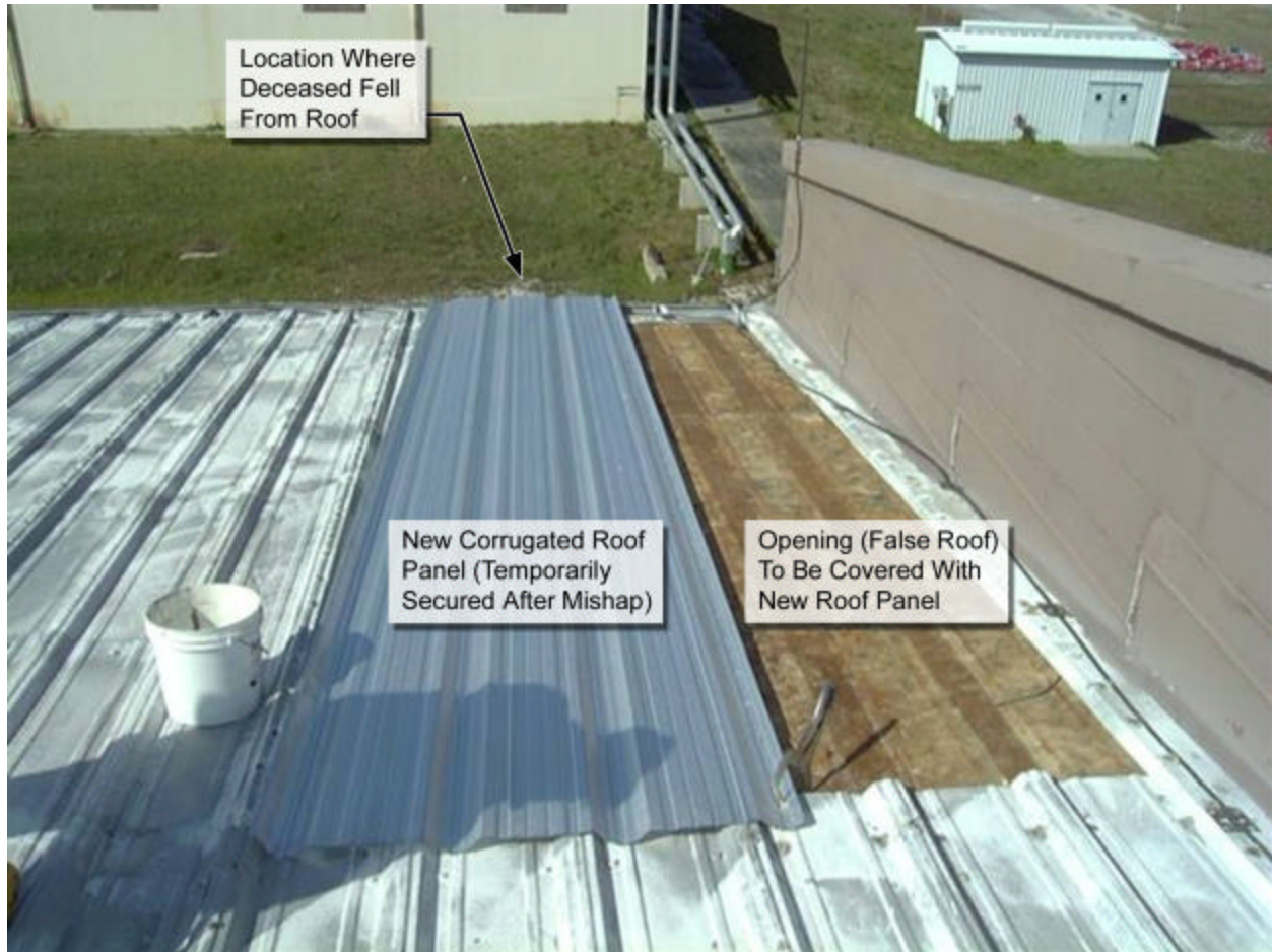
Figure 4. View of Mishap Location From Roof
